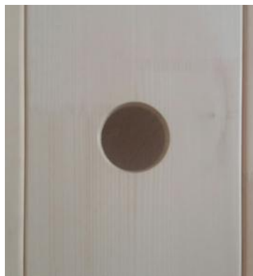
Fig. 38: Installing the control panel
