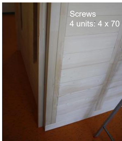
Fig. 46: Installation of the spacer strips of the rear wall
