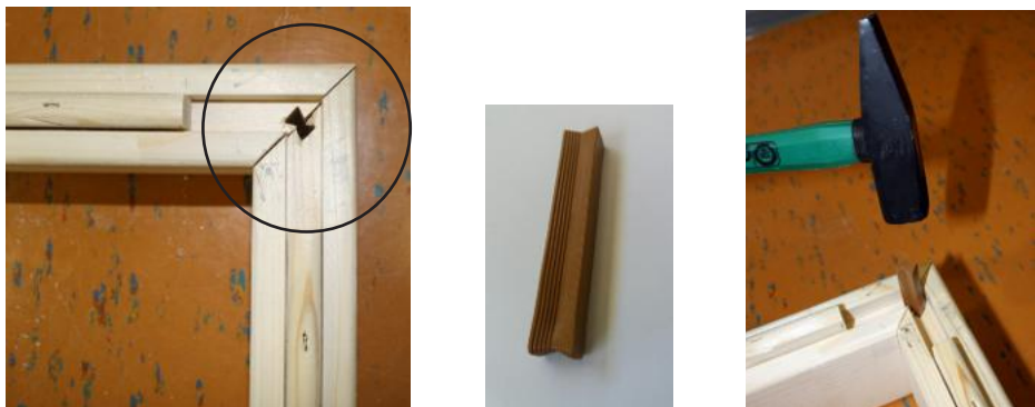
Fig. 2: Connect the floor frame elements
