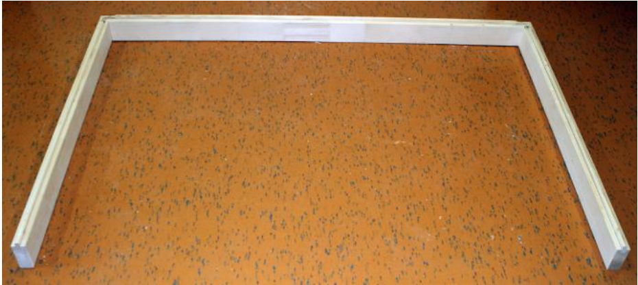
Fig. 1: Placing the three floor frame elements
