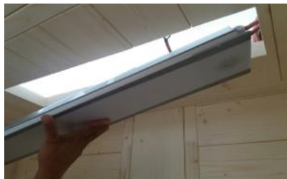
Fig. 44: Installing the colour light
