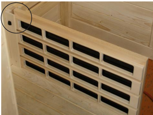
Fig. 32: Installation of the IR thermal plate VitaMy 164
