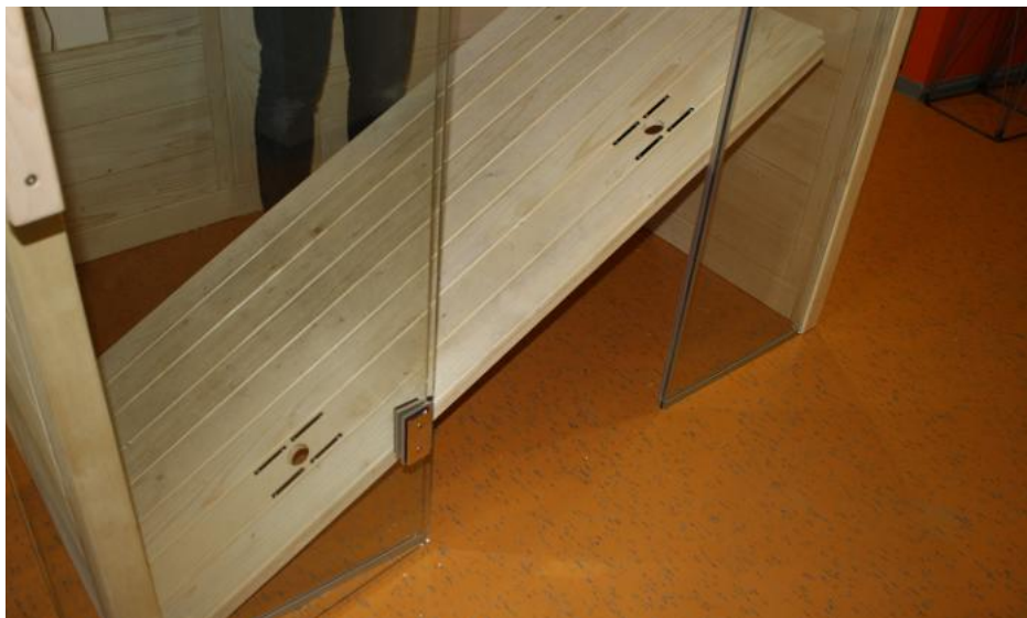
Fig. 26: Put the cabin floor in place
