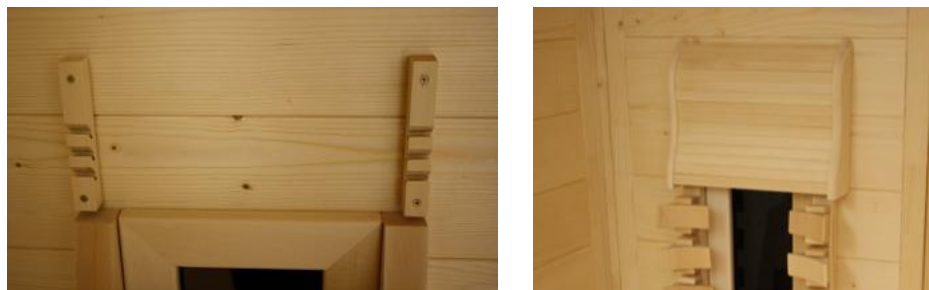
Fig. 47: Installation of the headrests
