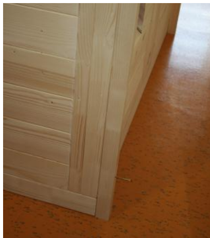
Fig. 46: Installation of the spacer strips of the rear wall
