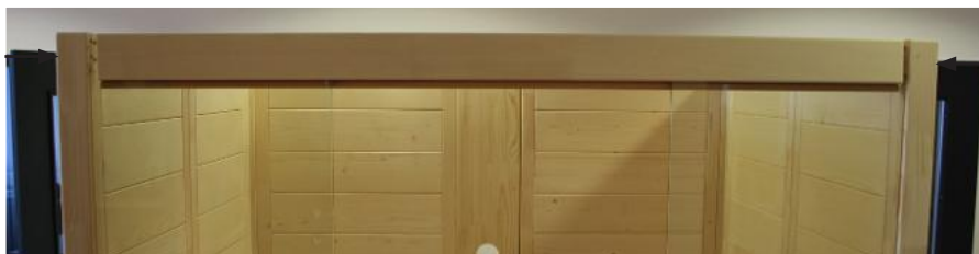
Fig. 13: Attaching the skirting
