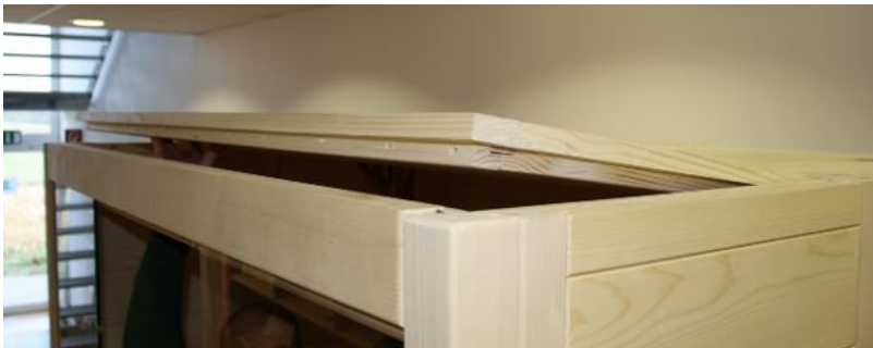
Fig. 17: Installing the roof element in the front
