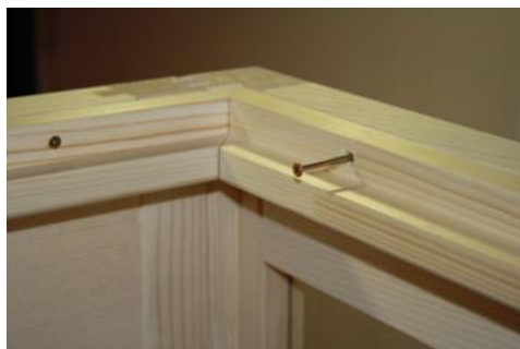
Fig. 14: Roof support slats installation
