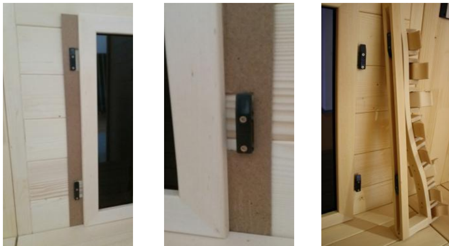
Fig. 48: Installing the backrests of the bench
