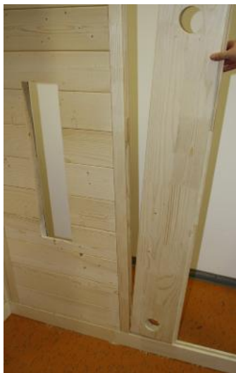
Fig. 6: Install the electrical element in place
