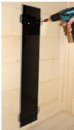
Fig. 36: Install the rear radiator (infrared radiator ECO 350)
